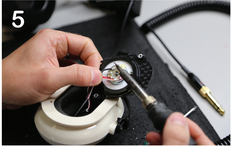
Using low heat (~600 deg), de-solder the existing leads from the driver
